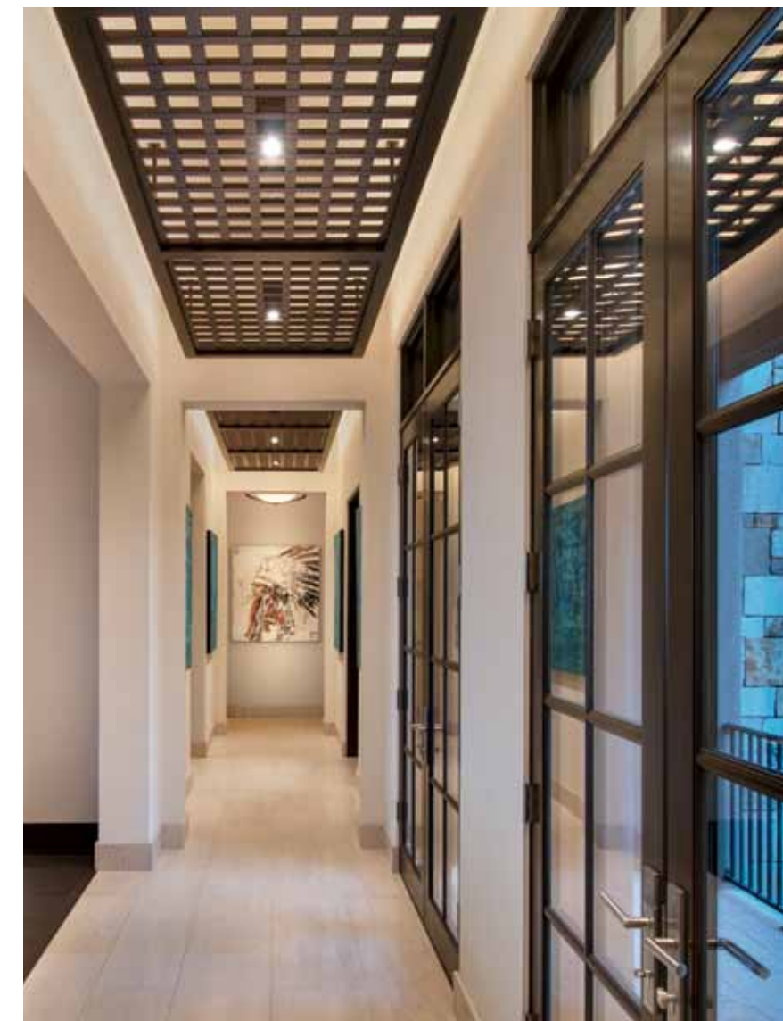
In lieu of traditional beams, the ceiling in the main hallway presents suspended backlit Lyptus wood grid panels. The grid was conceived by interior designer Janet Brooks and fabricated by Goodall Custom Cabinetry & Millwork; the honed limestone flooring is from Facings of America.
